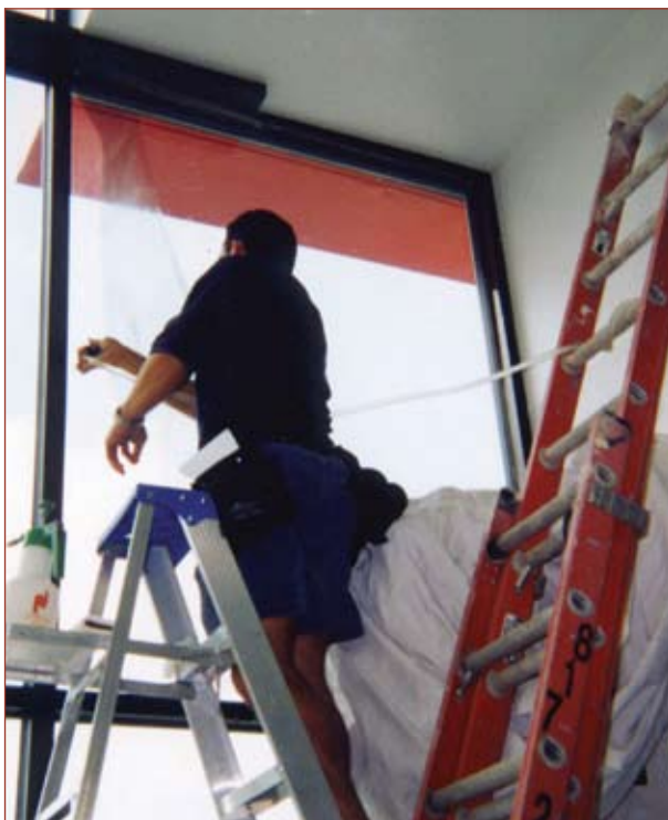
Security window film is an alternative to replacing existing glass with laminated glass. It can be applied to the interior surface of existing glass.
